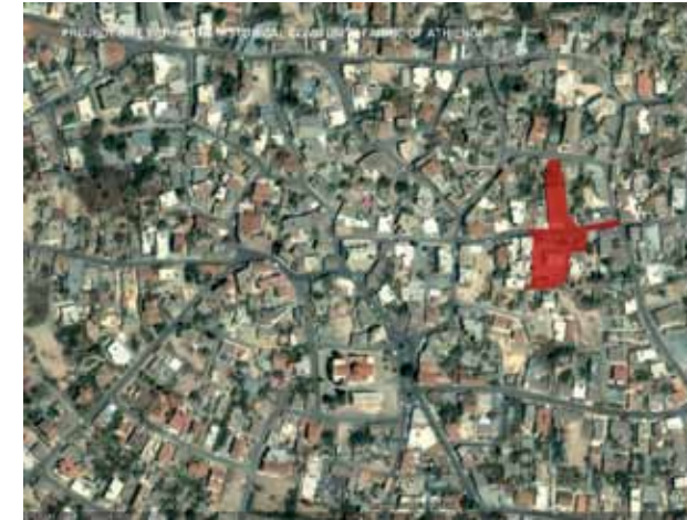
project site within Athienou community
