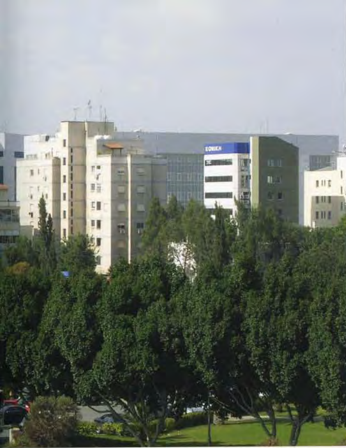
Detail tower surface
